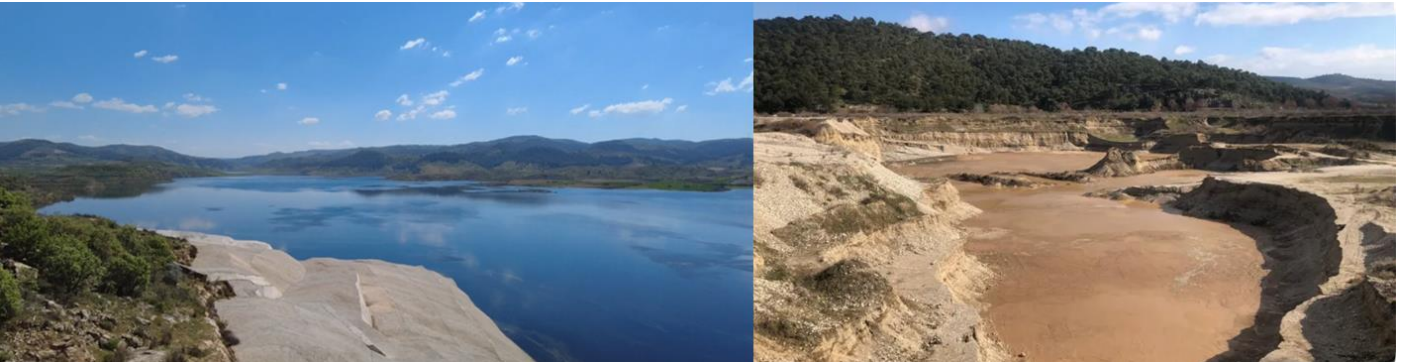
Figure 4 Gördes dam: shallow reservoir level (left) and siltation downstream of the dam (right)
