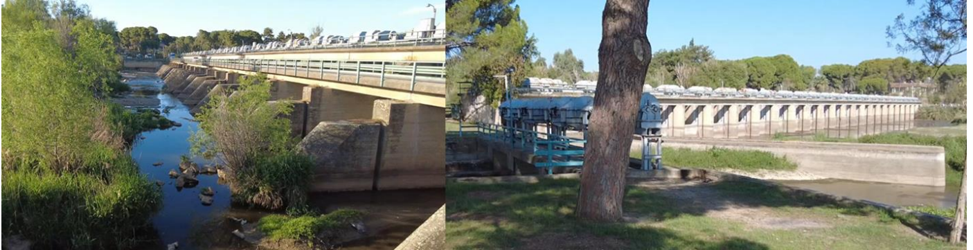
Figure 3 Ahmetli weir on the Gediz River
