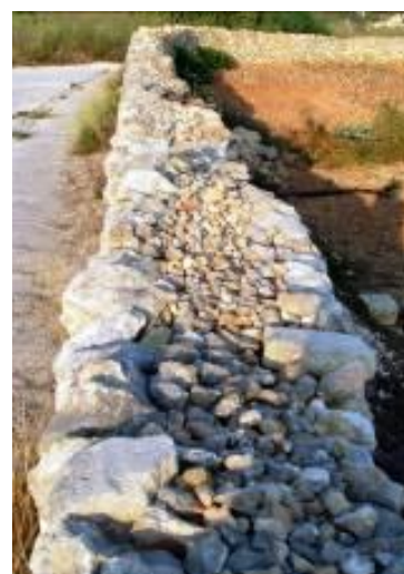
Rubble wall infill, 'mazkan' (Wied Ġhomor, Malta)
