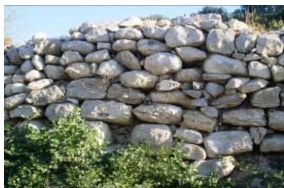
Rubble walls are 'dry' stone walls (Wied Qirda, Malta)
