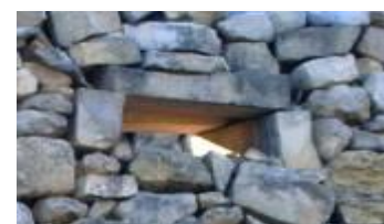
Flow hole at base of rubble wall (Wied Ġhomor, Malta)
